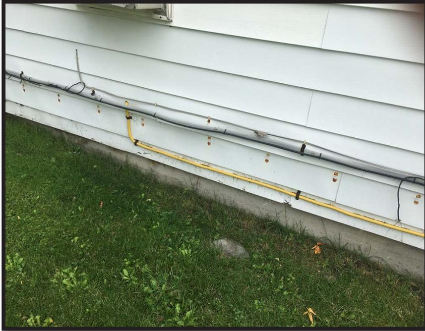
Flexible gas line used in an unprotected area
