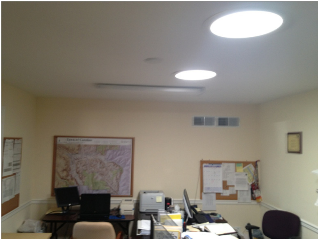
Building Interior with Sun Tube Lighting
