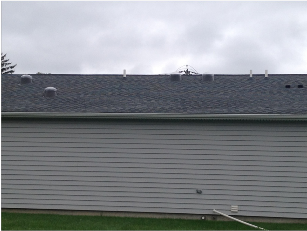
North Side of Building with Sun Tubes on the Roof
