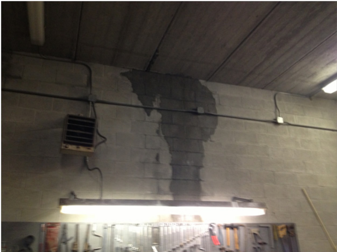
Continuous leak in the ceiling of the sewer plant
