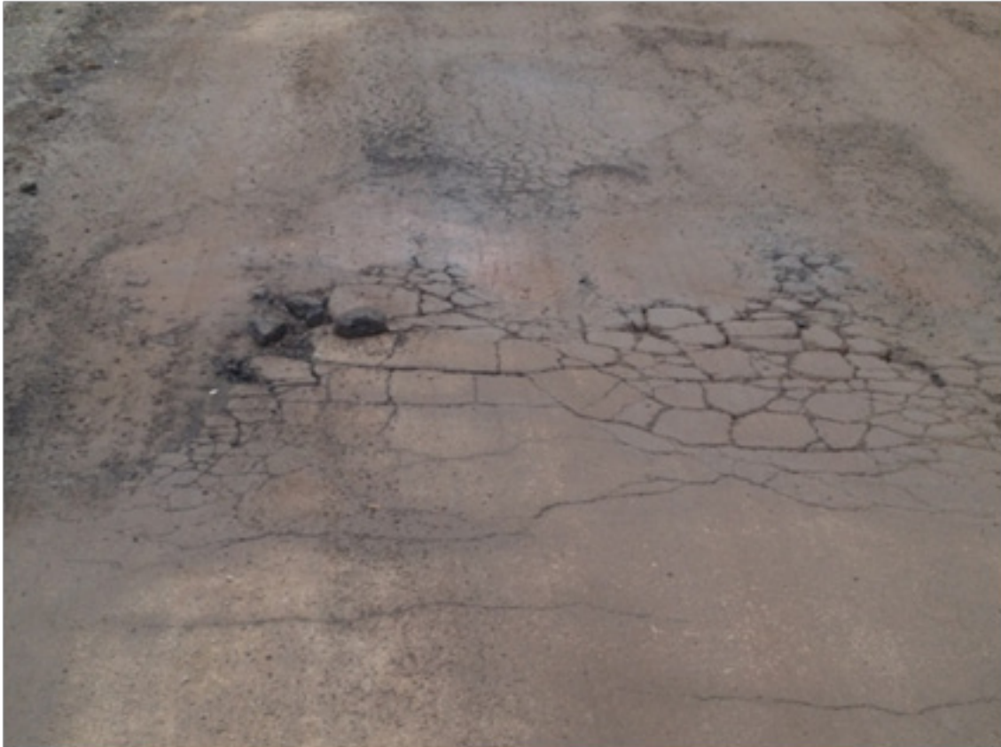
Cracks and pot holes in West Lake Street
