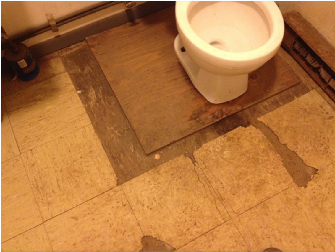
Hole in restroom floor covered by a piece of wood in the Department of Public Works building
