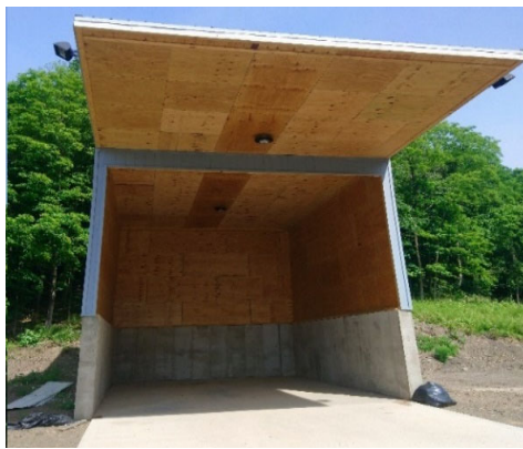
New Salt Shed (June 2021)
