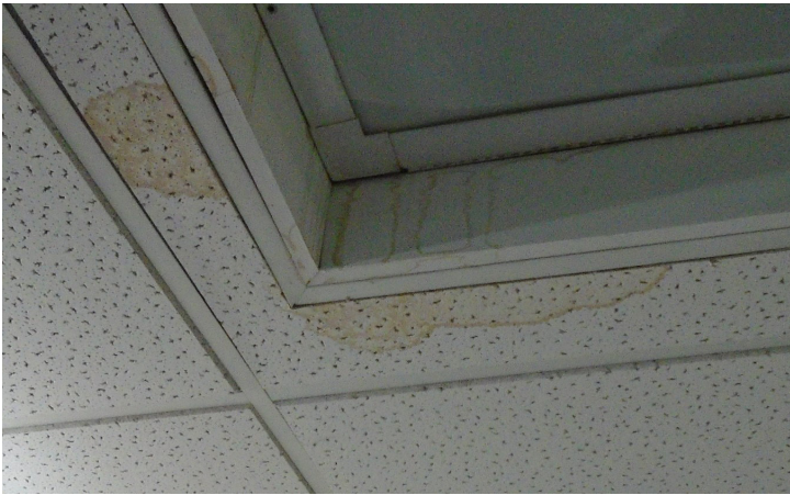
FIGURE 2: Water Leakage Above IT Assets
