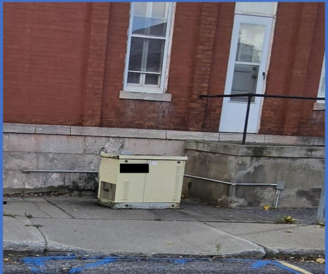
The level landing at the top of a curb ramp along the accessible route at a City's police facility was obstructed by a generator.
