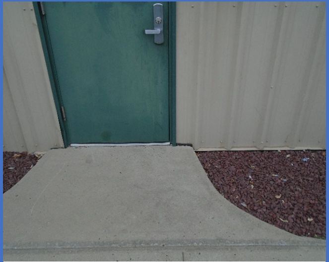
Not enough clearance on the latch side of the door to accommodate a wheelchair at a Town's recycling center.
