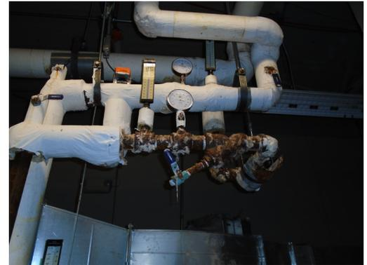
Picture 6 – Rusted pipe joint at JSHS building
