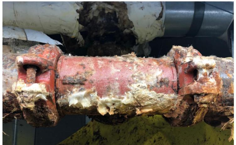
**Picture 3 – Rusted pipe joint at JSHS building**
