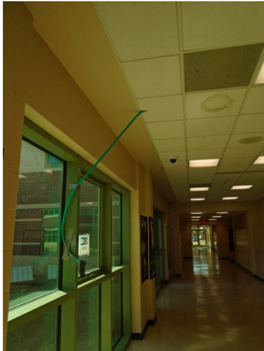
Picture 4 – Hose to catch leaks in JSHS hallway
