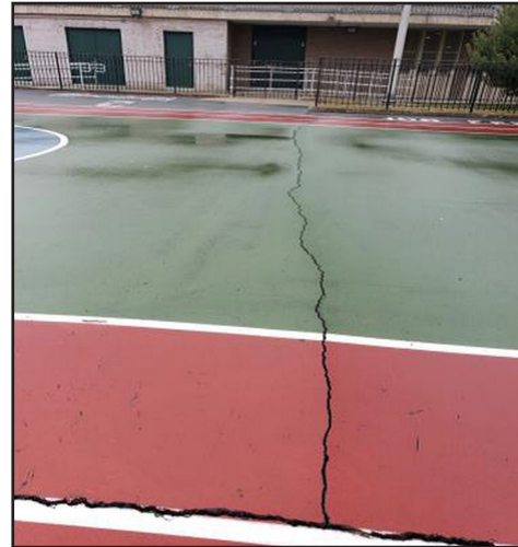
Image 6 (right): Cracked playground pavement. Image 7 (bottom left): Protruding nails/screws on safety mat. Image 8 (bottom right): Broken playground slide
