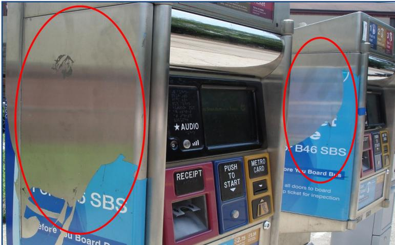
**Figure 4:** Damaged SBS bus stop signage with illegible statements.
