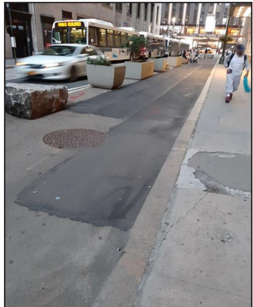
**Figure 4.** Photo of tan granular paint missing from pedestrian plaza.
