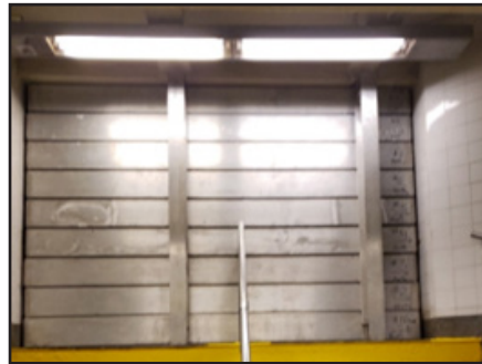
Figure 3 – Stop logs consist of a deployable set of watertight vertical metal logs that can be installed around station entrances to protect against water intrusion, especially where it is not feasible to install swinging or sliding doors. Whitehall Street Station 12/13/2021.
