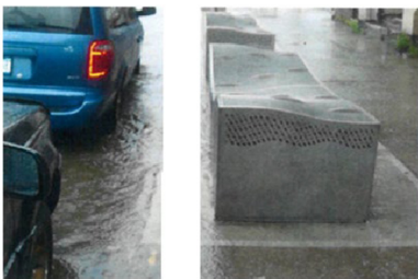
Fig. 1: Raised Ventilator / Streetscape Preventing Water Ingress during Storm Flooding
