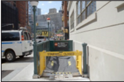
Figure 1 – A flex-gate is a permanently installed containment box within a staircase and a deployable fabric cover, which can be locked in place when a storm event occurs. Franklin Street Station #1.
