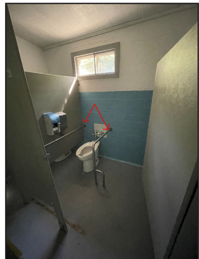
Figure 1 – Examples of potential improvement areas identified in restrooms (clockwise from upper left): stall too narrow for wheelchair turnaround (Allegany State Park); stall with missing rear grab bar and grab bar obstacle to wheelchairs on either side (Jones Beach State Park); stall with missing rear grab bar and grab bar obstacle to wheelchairs (James Baird State Park); restroom not wheelchair accessible (Letchworth State Park); lack of wheelchair-accessible stall (Taconic State Park).
