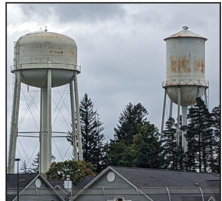
Water towers found at Sunmount Developmental Disabilities Services Office.
