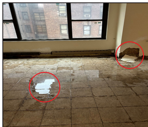
Figure 5 – Peeling paint and water leak in a commercial space at Findlay House (February 6, 2025).
