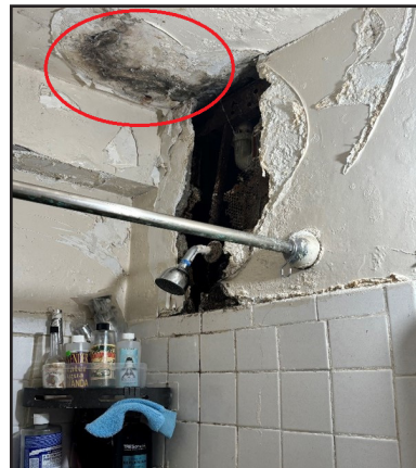
Figure 3 – (above) Mold on a ceiling; (left) hole in bathroom wall and peeling paint in occupied Classon unit (February 5, 2025).
