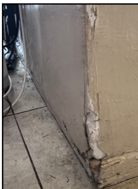
Figure 9 – Cracks on living room wall
