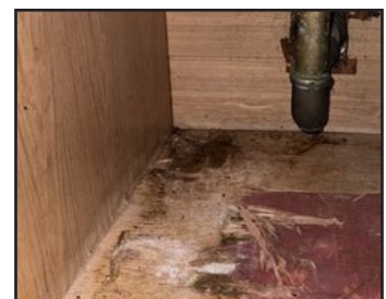
Figure 17 – Possible mold under the kitchen sink
