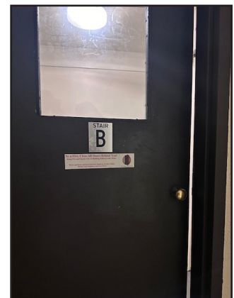
Figure 13 – 10th-floor fire door of Stairwell B does not self-close and latch
