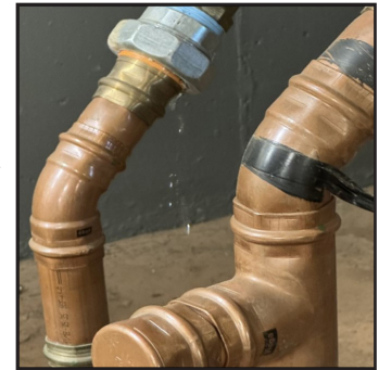
Figure 15 – Leak in boiler room
