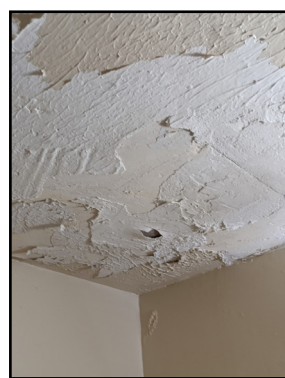
Figure 11 – Peeling paint on bathroom ceiling
