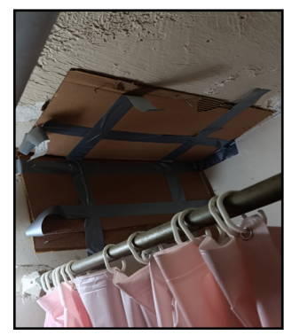
Figure 12 – Hole in bathroom ceiling covered with cardboard
