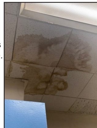
Figure 1 – Water-damaged ceiling tiles in closet
