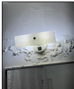
Figure 10 – Bubbled paint/plaster on bathroom wall
