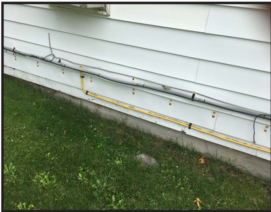
Flexible gas line used in an unprotected area (Relax Inn Motel, Watertown, Jefferson County DSS)
