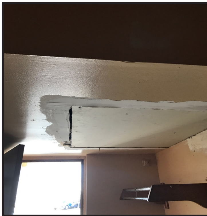
Water damage to ceiling in room with improper repair (Plantation Motel, Island Park, Nassau County DSS)
