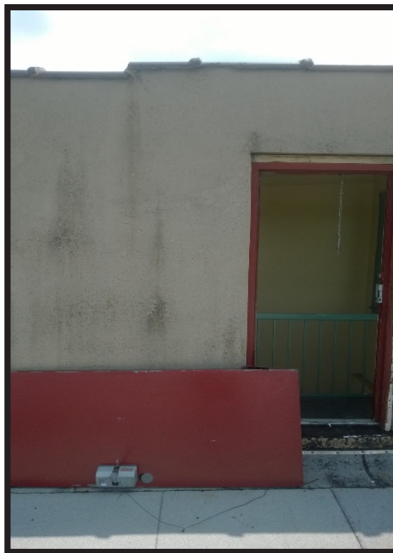
Detached door allowing unsecured roof access (Community Housing Innovations family shelter, Westchester County)
