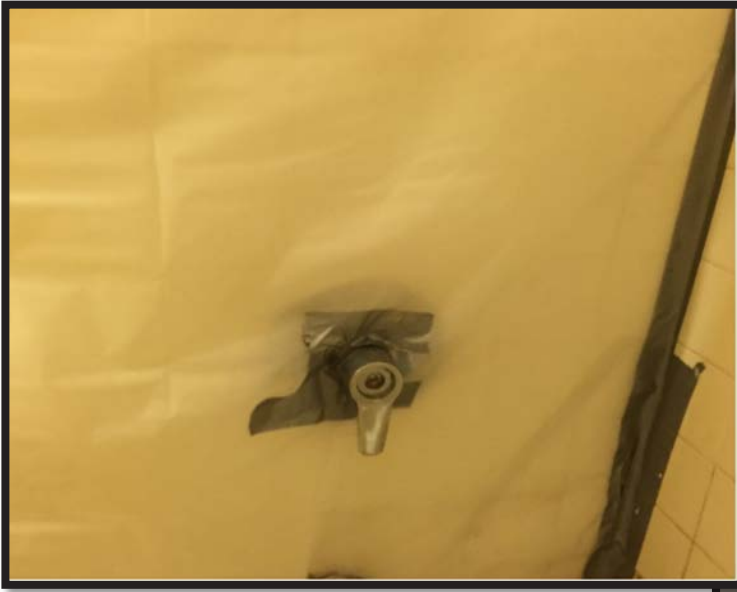
Shower fixture/wall repaired with heavy-duty plastic sheeting and duct tape (St. John's Place family shelter, Brooklyn)
