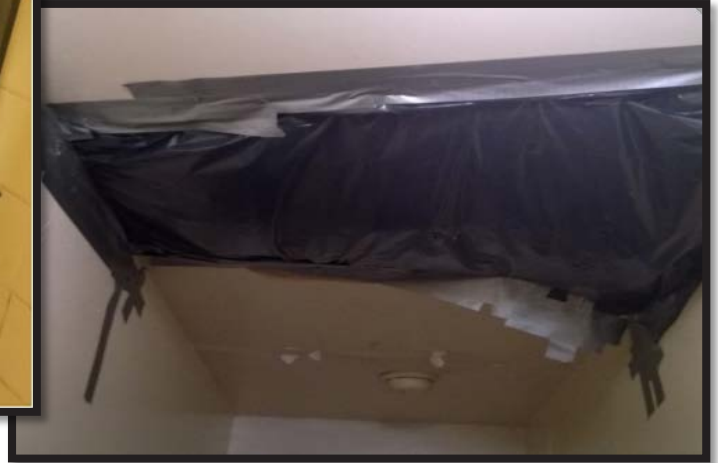
Trash bag and duct tape ceiling repair (Jennie A. Clarke family shelter, Manhattan)
