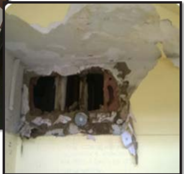
Wall with water damage and unrepaired hole (Kingsboro Psychiatric Center, Building 8 men's shelter, Brooklyn)
