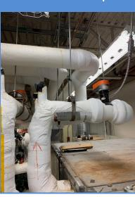
Repairs made to pipes adjacent to air handler AHU #13
