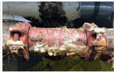
Picture 3 – Rusted pipe joint at JSHS building
