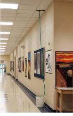
Picture 2 – Hose and bucket to catch leaks in JSHS hallway
